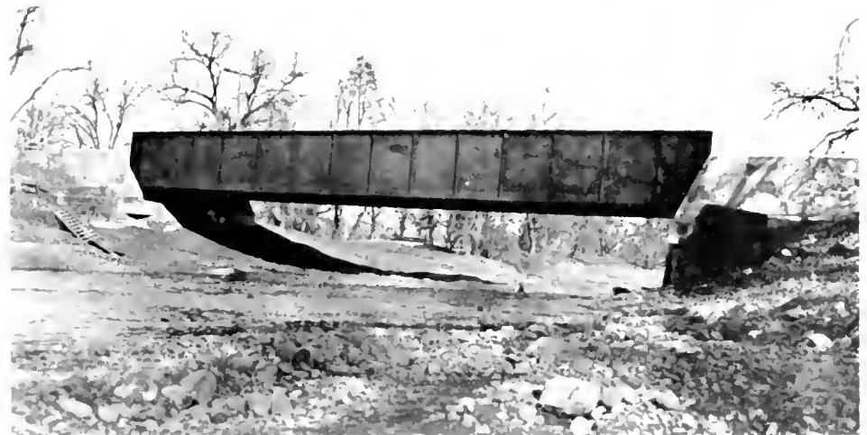
Single span steel railroad bridge State was able to buy for replacement
